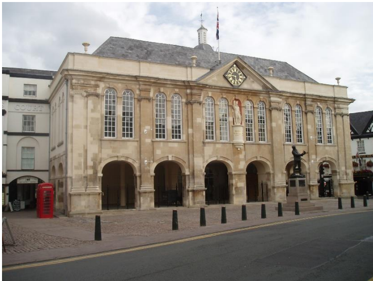
Figure 29 - Shire Hall, Monmouth
